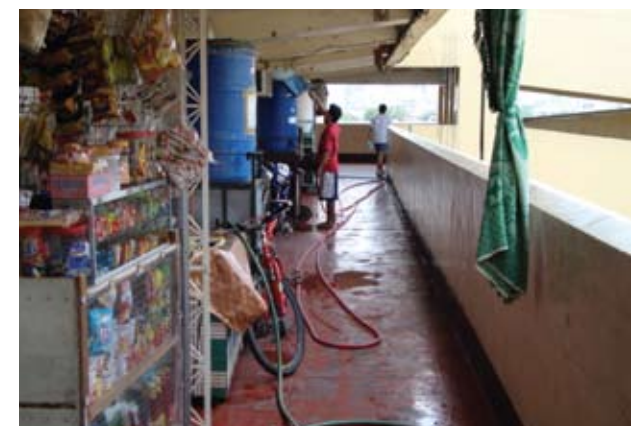
Providing water services to an apartment block in Punta, Sta. Ana, Manila, Philippines.
