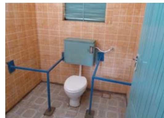
A toilet designed for disabled users in the public sanitation facility constructed by the Nanyuki Water and Sewerage Company, Nanyuki, Kenya.
